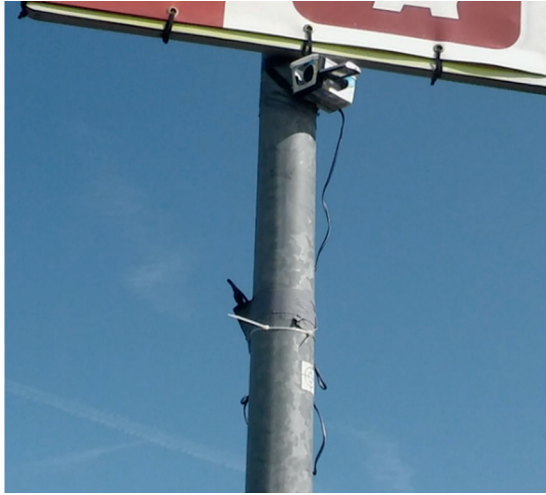
Fig. 2. Camera recording traffic movements over the roundabout
